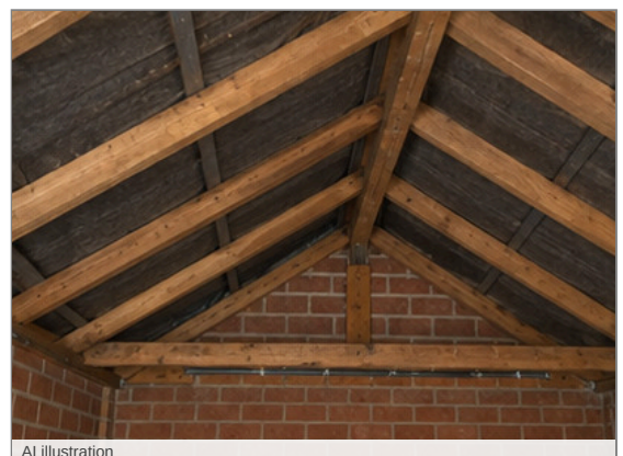
Photo - 97 Roof structure
