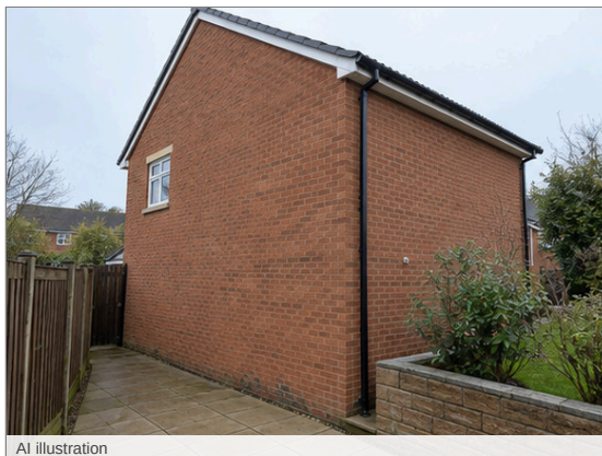
Photo - 22 Left elevation - high ground level
