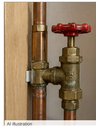
Photo - 76 Internal stop valve
