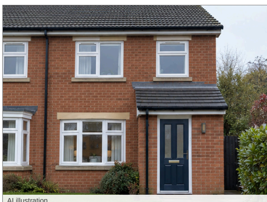
Photo - 23 Front windows
