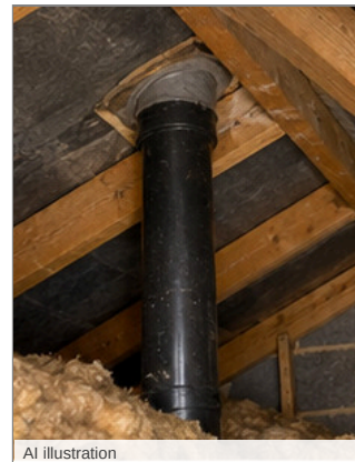
Photo - 92 Soil vent pipe visible in the loft
