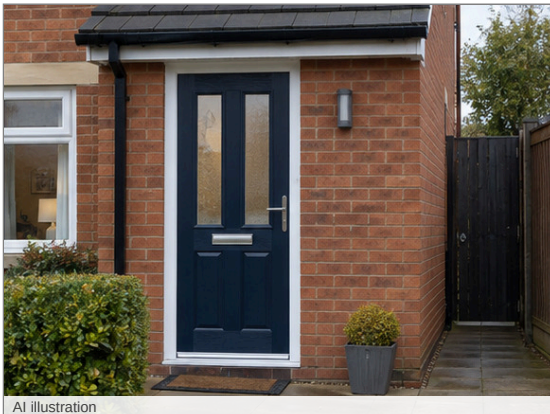
Photo - 26 Front door
