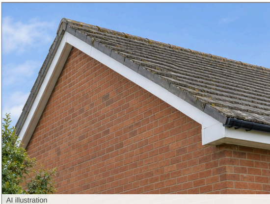
Photo - 7 Rear right verge
