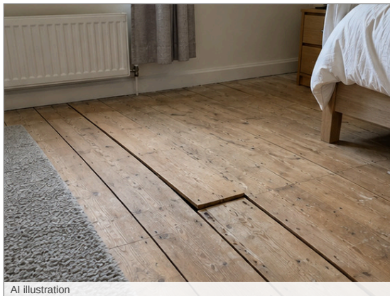
Photo - 44 Rear bedroom - loose floorboards
