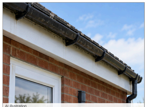
Photo - 17 Rear gutter
