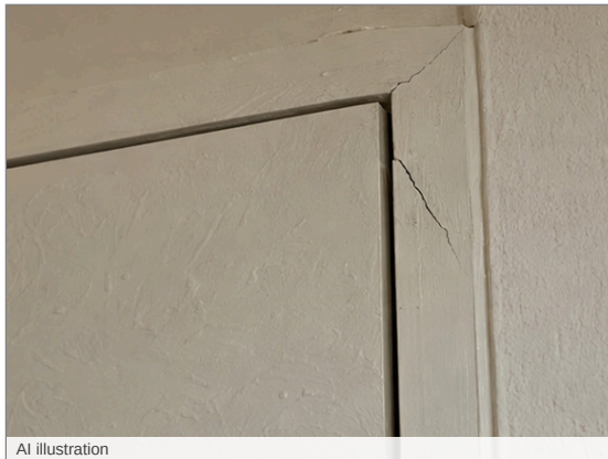
Photo - 43 Front bedroom cupboard - minor fracture noted
