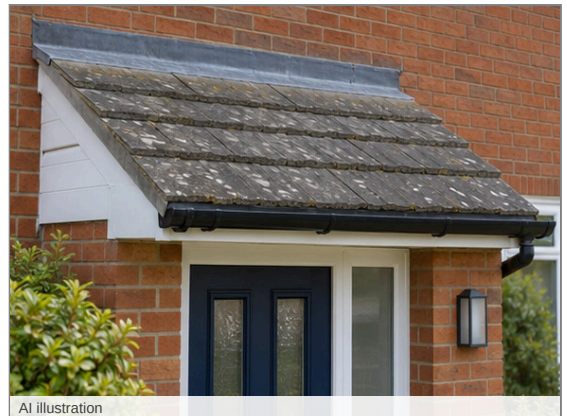
Photo - 8 Main entrance roof
