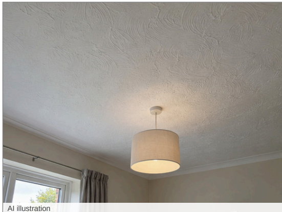
Photo - 39 Typical ceiling
