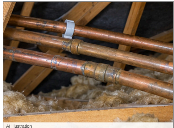
Photo - 84 Uninsulated water pipework in the loft
