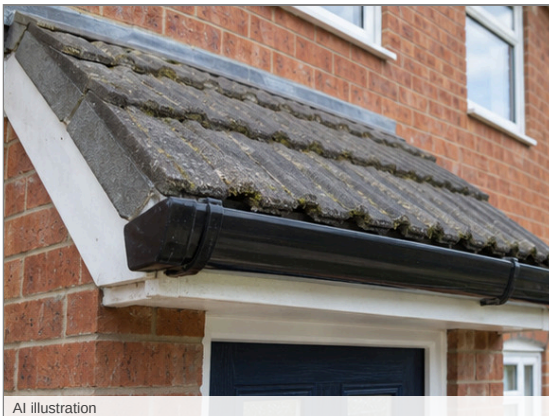
Photo - 14 Main entrance roof gutter
