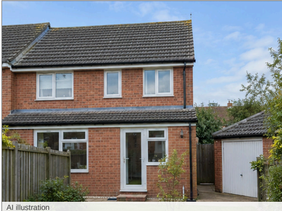
Photo - 11 Rear roof slope
