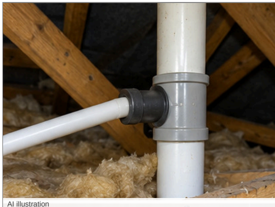
Photo - 83 Boiler condensate connected to soil vent pipe
