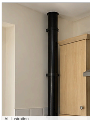
Photo - 93 Soil vent pipe visible in the kitchen
