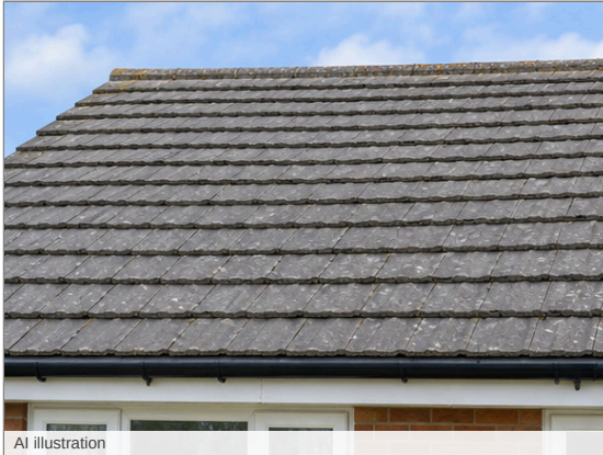
Photo - 5 Front roof slope
