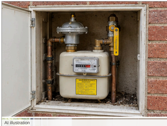
Photo - 70 Gas meter and shut off valve
