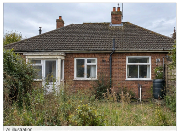
Photo - 33 Rear elevation
