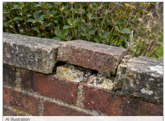
Photo - 127 Loose masonry
