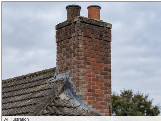
Photo - 7 Rear-right chimney stack
