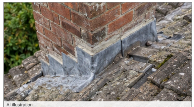
Photo - 10 Rear-right chimney stack - drone view
