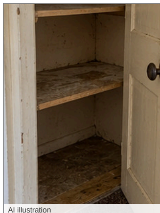
Photo - 98 Entrance hall cupboard
