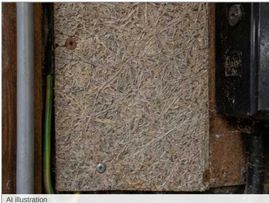
Photo - 103 Potential asbestos containing material
