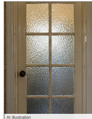
Photo - 92 Typical glazed door
