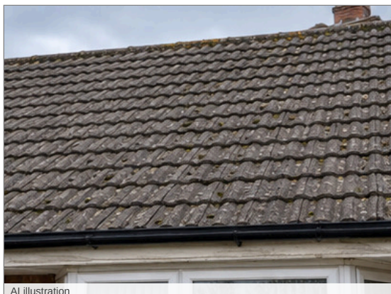
Photo - 12 Front roof slope
