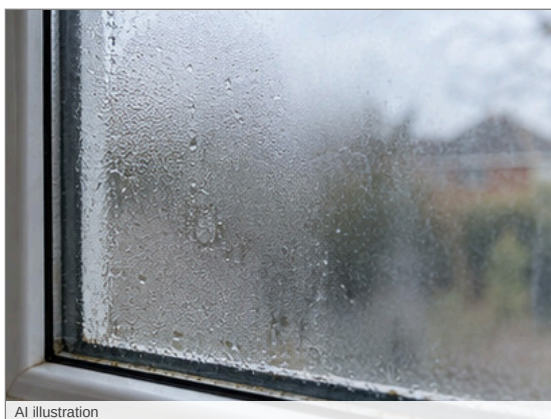
Photo - 40 Failed double glazing
