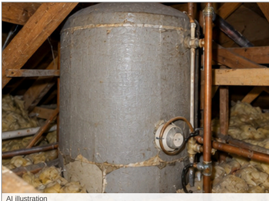
Photo - 120 Hot water cylinder
