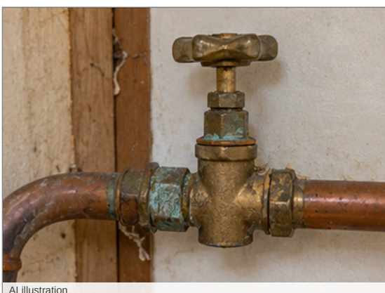
Photo - 110 Internal stop valve
