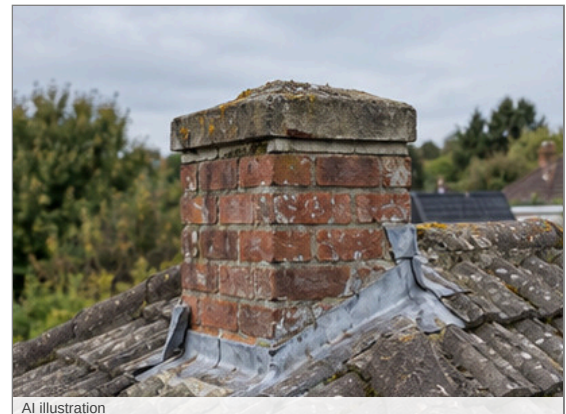
Photo - 8 Rear-left chimney stack
