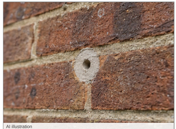
Photo - 31 Evidence of injected insulation
