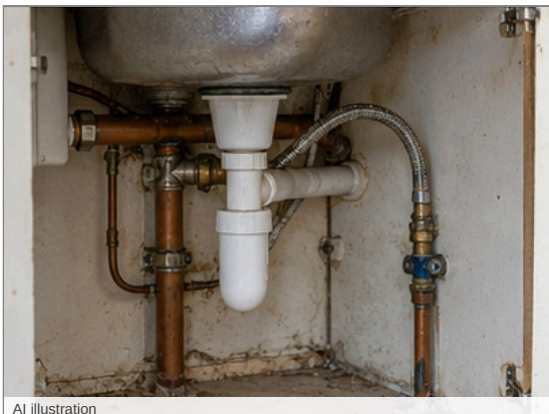
Photo - 108 Under sink cupboard
