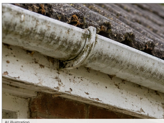
Photo - 21 Front gutter
