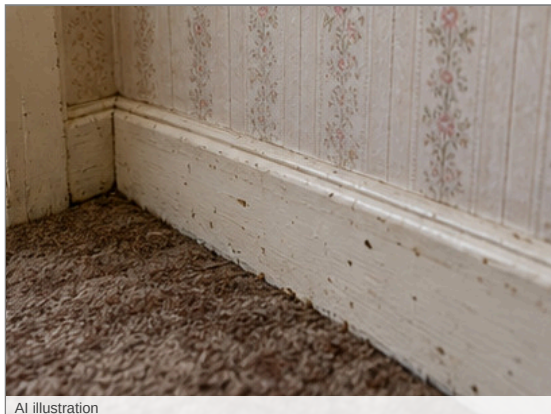
Photo - 91 Skirting board
