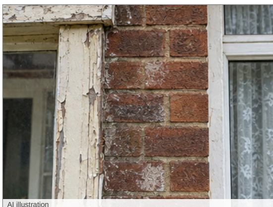
Photo - 32 Front cladding
