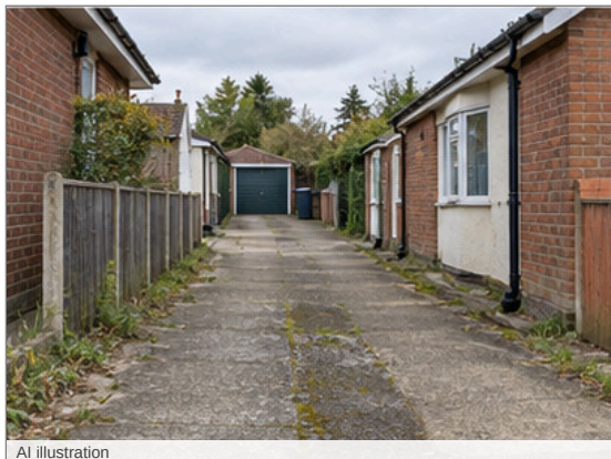
Photo - 132 Shared driveway
