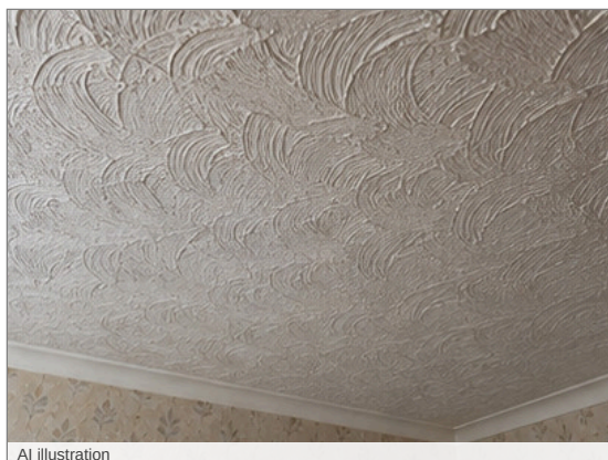
Photo - 67 Typical textured ceiling
