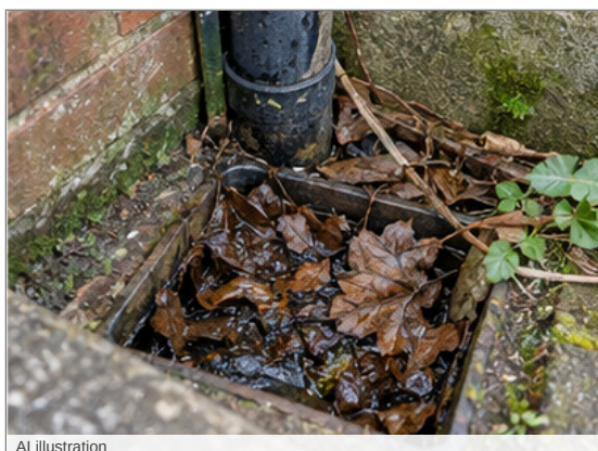
Photo - 125 Rear left downpipe gully blocked
