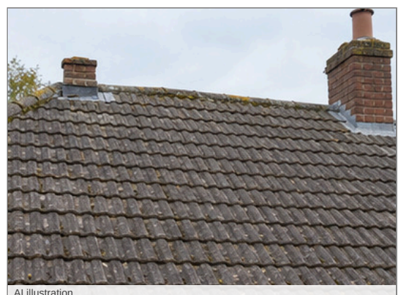
Photo - 15 Rear roof slope
