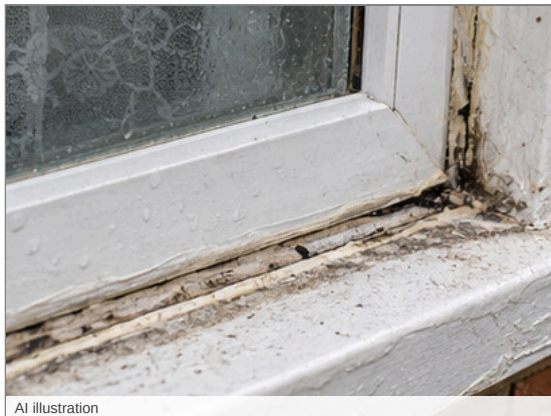
Photo - 38 Replace sealant
