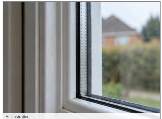
Photo - 39 Thin double glazing
