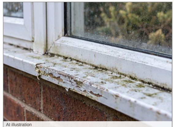
Photo - 90 Typical sill
