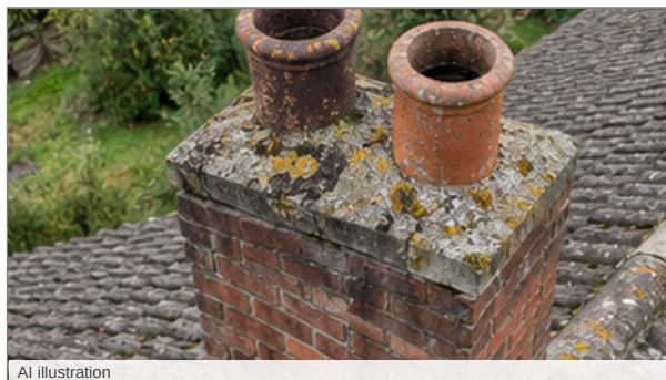
Photo - 9 Rear-right chimney stack - drone view
