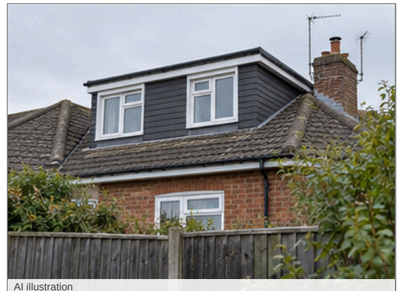
Photo - 133 Neighbours loft conversion
