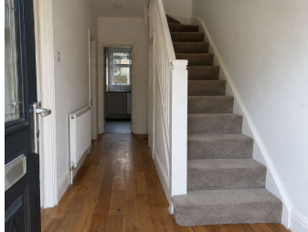
P1 Entrance hall and stair turn A1/A2 (illustrative image)
