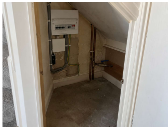
P3 Under-stairs consumer unit S1 and stopcock S2 (illustrative image)
