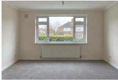
P2 Living-room window W2 and radiator (illustrative image)
